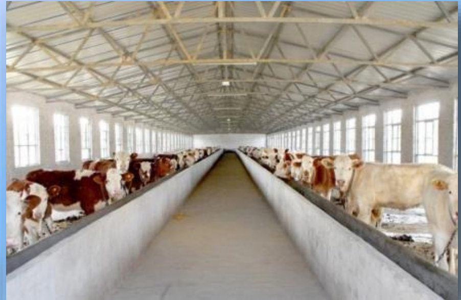
Livestock Feeding Shed
